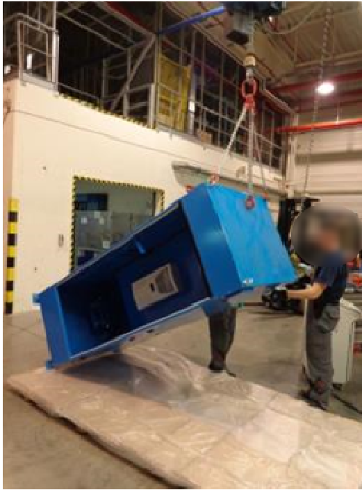
Figure 14: Cabinet lifting process using the rings
